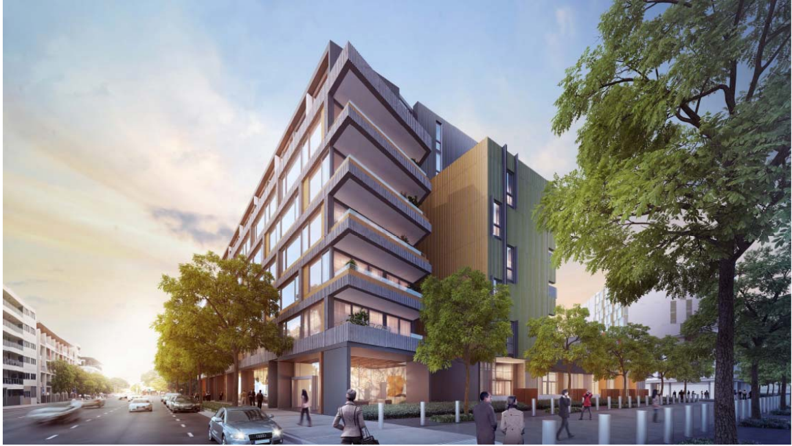
Figure 10: Photomontage of Building D as viewed from corner of Epsom Road and proposed Fuse Street facing west (Stage 1)
