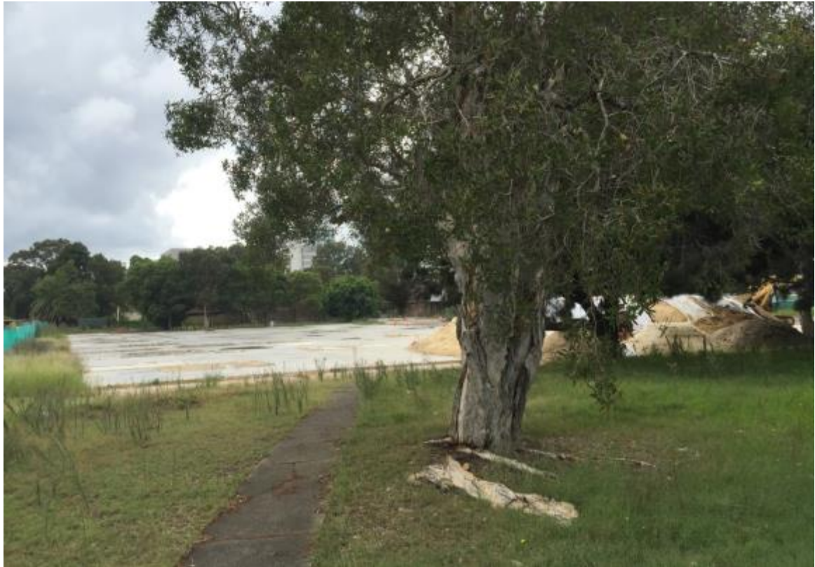
Figure 5: Site viewed from Epsom Road facing north east
